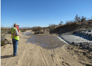
Recharge Capacity is 1,500 Acre Feet Per Year. An Acre Foot Would Cover a Football Field One-Foot Deep.
